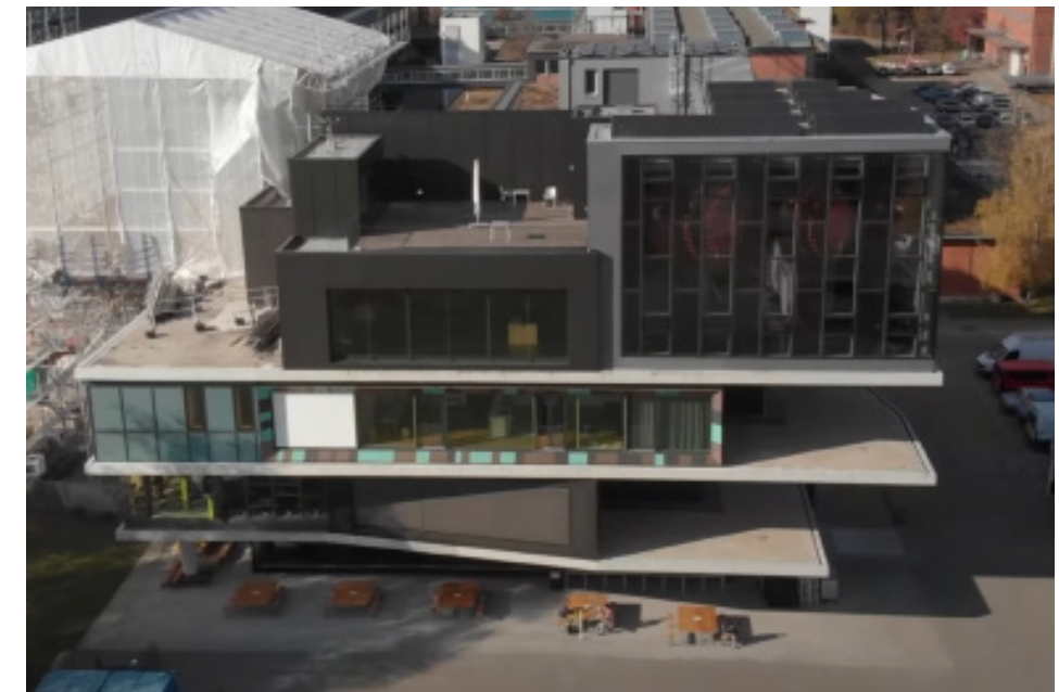
NEST building Source: EMPA youtube channel
