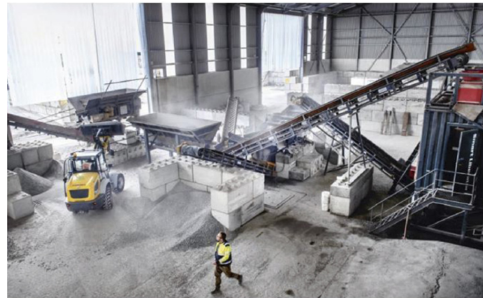
SmartCrusher installation, NL
