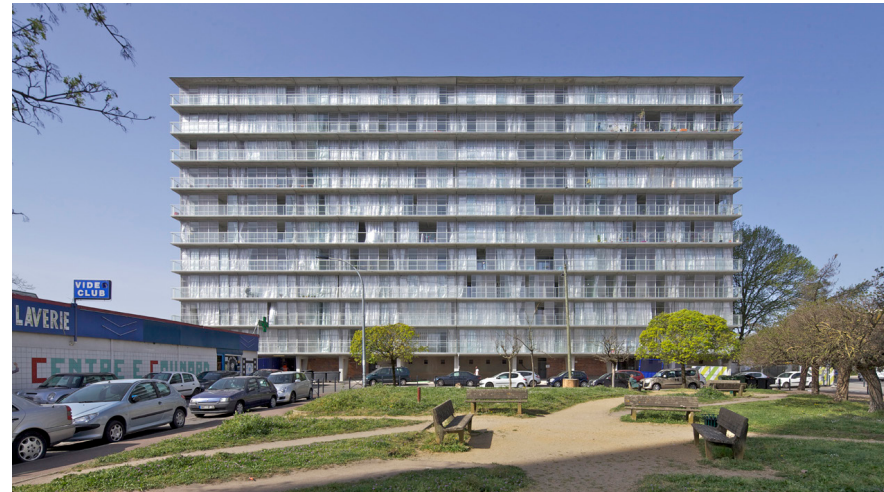
New facade. Soucre: Lacanton Vassal
